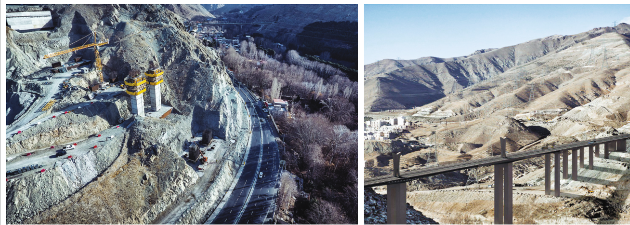
Construction of Karaj Northern Highway (EPCF)
