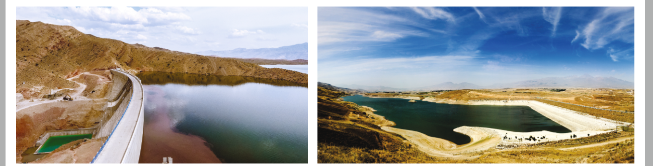
Yamchi (Ardebil) Reservoir Dam
