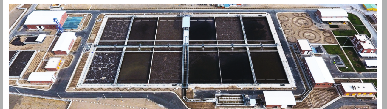
Construction Operation, Procurement & Installation of Electro Mechanical Equipment, Instrumentation of Ardabil Sewage Treatment Plant.
