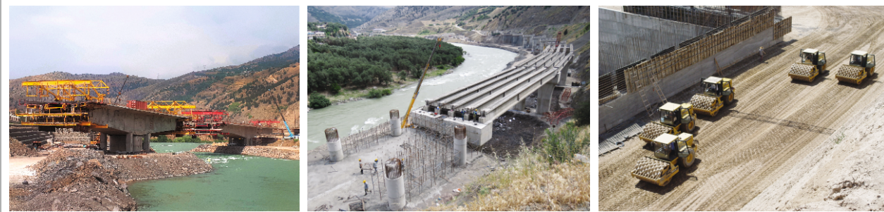
Construction of Manjil to Roudbar Highway
