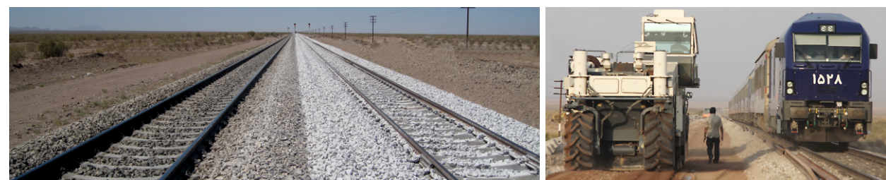
Rehabilitation of Tehran - Shahrood railway 30km
